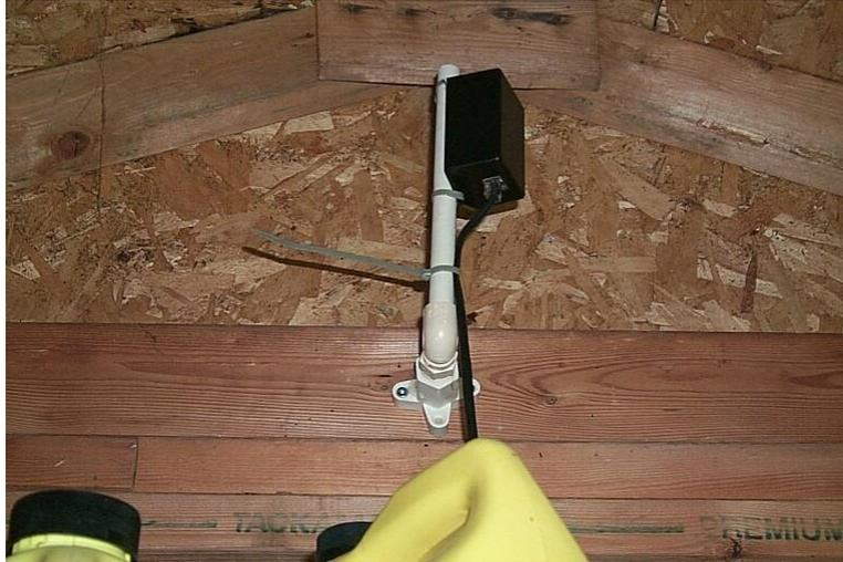
Here an antenna is mounted in a shed using PVC plumbing hardware purchased at a local hardware store. The antenna is attached using nylon cable ties.
